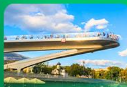
Floating Bridge Moscow
